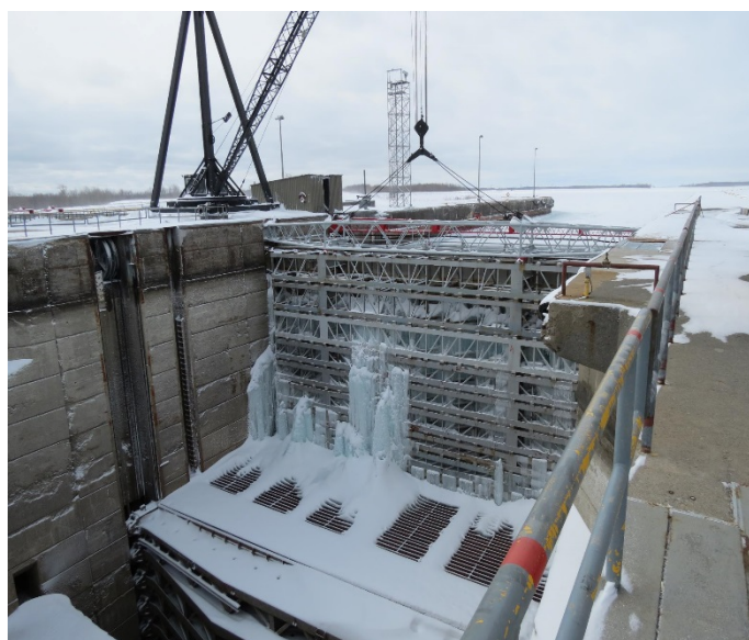
Figure 10: Winter Lock Maintenance (Source: SLSDC Facebook Page)
