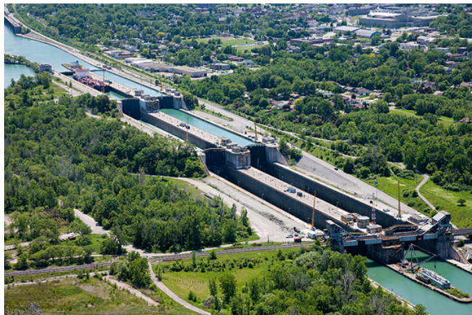
Figure 9: Welland Canal Locks 4, 5 & 6 (Source: SLSMC)
